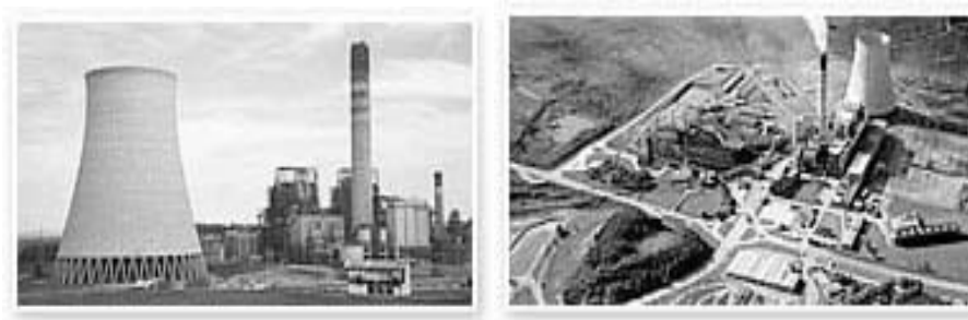
Figure 1 The Usina Presidente Médici Power Plant, southern Brazil
